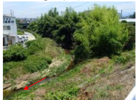
④中庄橋下流
