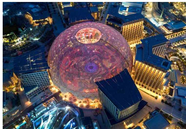
Al Wasl Plaza ©Expo 2020 Dubai LLC - SO
