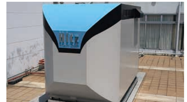
Commercial and Industrial Fuel Cell (Solid Oxide Fuel cell or SOFC)
