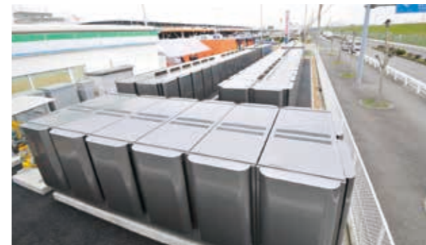
Fuel cell system of 1.2 megawatt solid oxide fuel cell(or SOFC) The service started in March 2015
