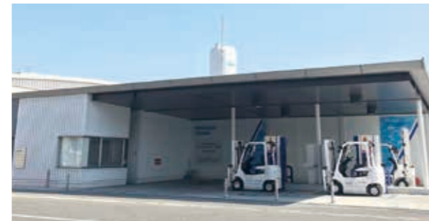
Hydrogen supply facility for industrial vehicles (Opened in March 2017)
