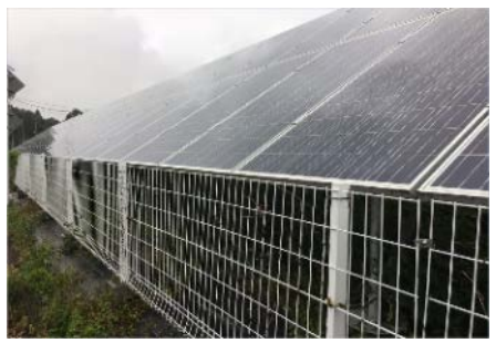
(不適切な柵塀設置の事例)
